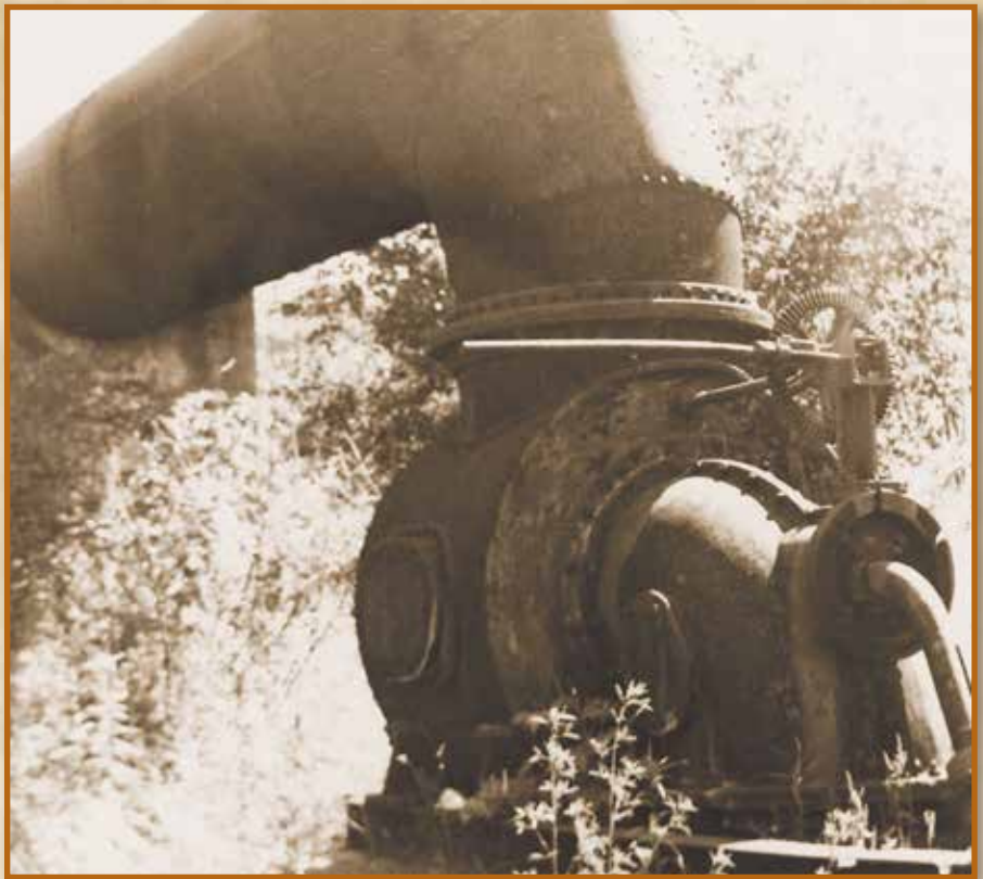
Power was generated by pushing water through this intake valve.
