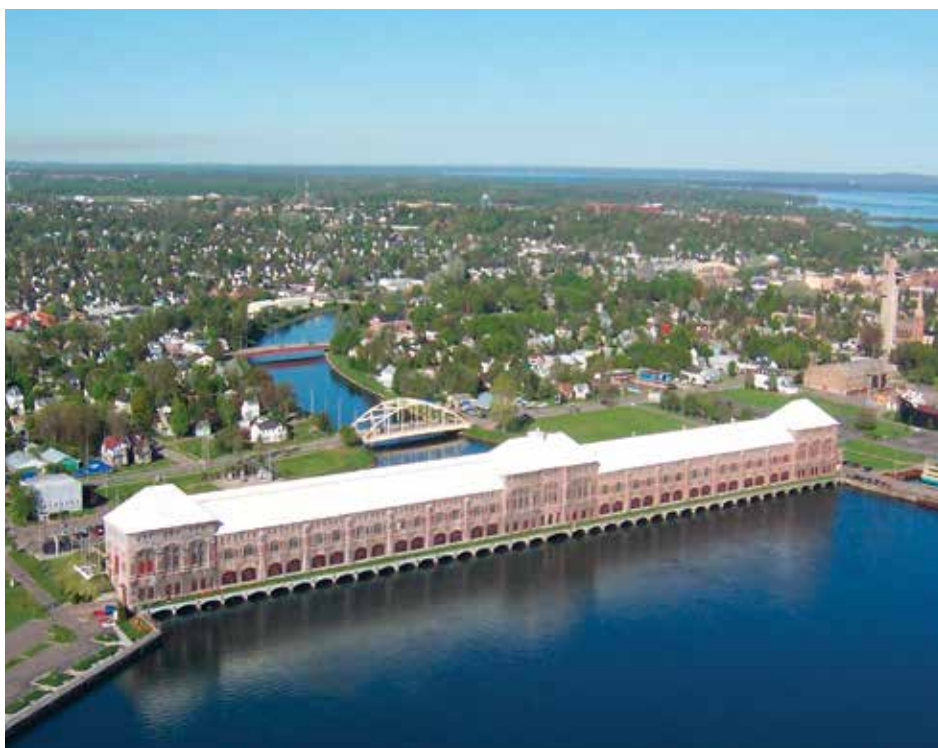
Cloverland Electric Cooperative's hydroelectric plant in Sault Ste. Marie generates between 25 and 30 megawatts of electricity. Clean, renewable hydro makes up nearly 35 percent of the co-op's fuel mix. To see a recent chart showing what your electric co-op's fuel mix is, visit countrylines.com and click on the co-op name and then click the Sept. 2013 issue.
