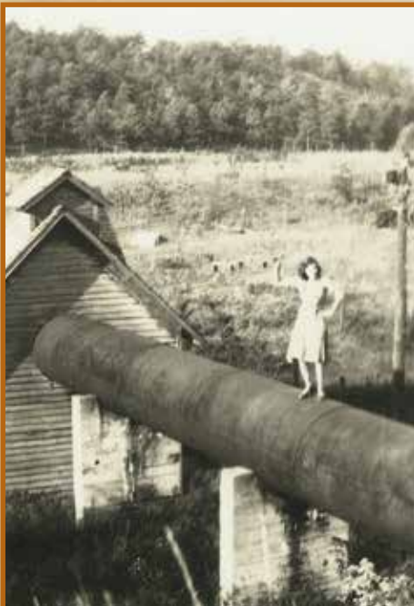
A young woman stands on the penstock intake valve that delivered water to the turbine for generating electricity.
