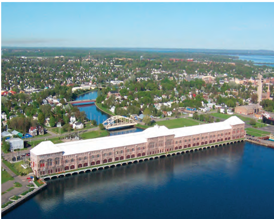
Cloverland Electric Cooperative's hydroelectric plant in Sault Ste. Marie generates between 25 and 30 megawatts of electricity. Clean, renewable hydro makes up nearly 35 percent of the co-op's fuel mix. To see a recent chart showing what your electric co-op's fuel mix is, visit countrylines.com and click on the co-op name and then click the Sept. 2013 issue.
