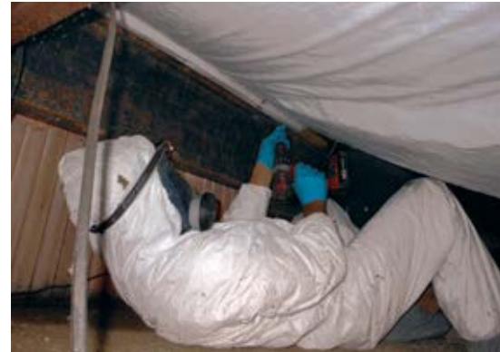
Fig. 2—Underneath the home, a "sling-patch" can be screwed into the inner side of the I-beam. It stretches to the other I-beam and holds insulation under the ductwork in place.
