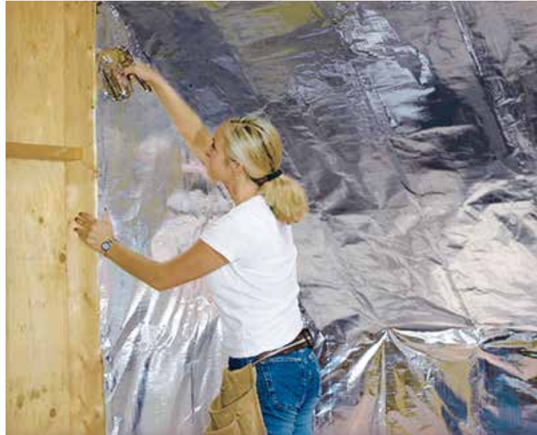
To install a radiant barrier, you will need a hand construction stapler, utility knife, and a long straight edge.
