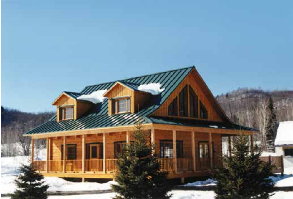
The metal roof on this log home features a standing seam design that reflects the sun's rays, making it both easier to cool in summer and great for shedding snow.
