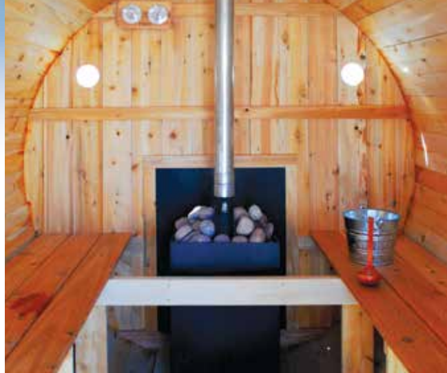
The cozy barrel sauna holds four adults comfortably and comes with a custom-fabricated woodstove, solar lights, a thermo-hygrometer, water pail, and a cedar spoon. The stove rocks all come from the U.P.
