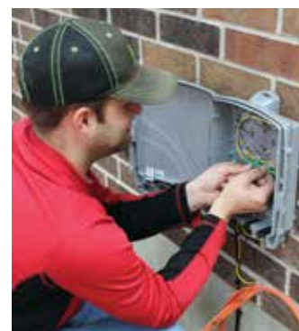
Tim Brown, installation and maintenance technician, installs an outdoor ONT at the home of a new fiber customer. Midwest Connections has more than 500 customers now surfing the web at previously unknown speeds.
