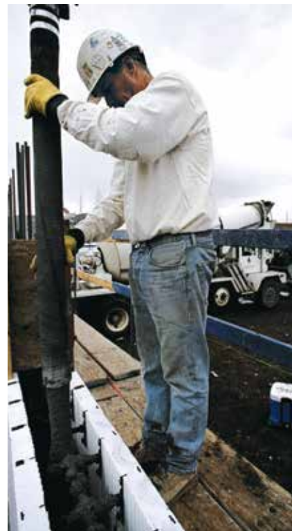
With “stay-in-place” construction, once the insulated forms are erected and reinforced steel installed, the concrete is pumped in from the top.
