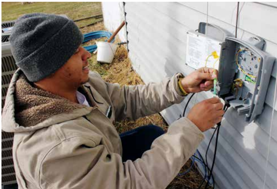
Joe Alford, installation and maintenance technician for Midwest Connections, connects fiber cable to the Optical Network Terminal.
