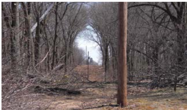
The ground-to-sky approach to line clearance helps to make sure that trees don't form a canopy over the lines.
