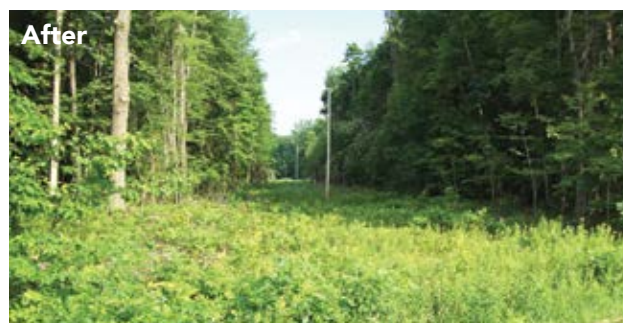
Before and after shots of a line circuit in Dowagiac. A newly cleared right-of-way can look extreme at first, but as the growth returns the landscape regains its natural beauty.
