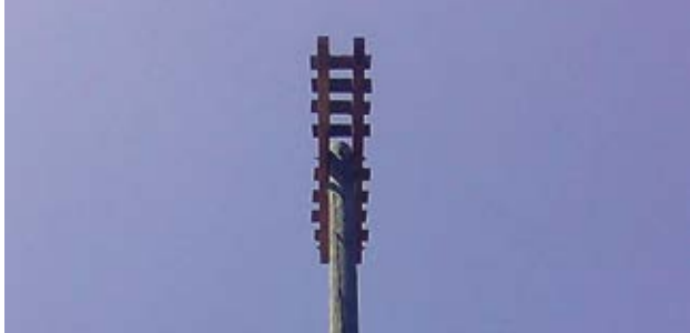
Blanchard lineman Jon Karcher built this osprey platform to coax the birds to nest away from our lines.
