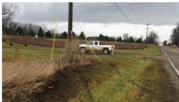
A recent car-pole encounter left the guy wire bent; when crews went to replace it, they found the pole was also broken.
