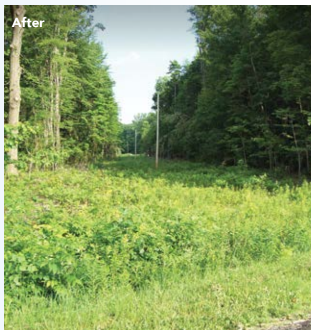
The ground-to-sky approach to line clearance helps to make sure that trees don't form a canopy over the lines.
