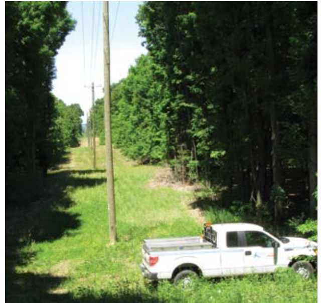
Great Lakes Energy uses the right-of-way to build and maintain its power lines and to manage trees and other vegetation within it that could pose a threat to your electric service.
