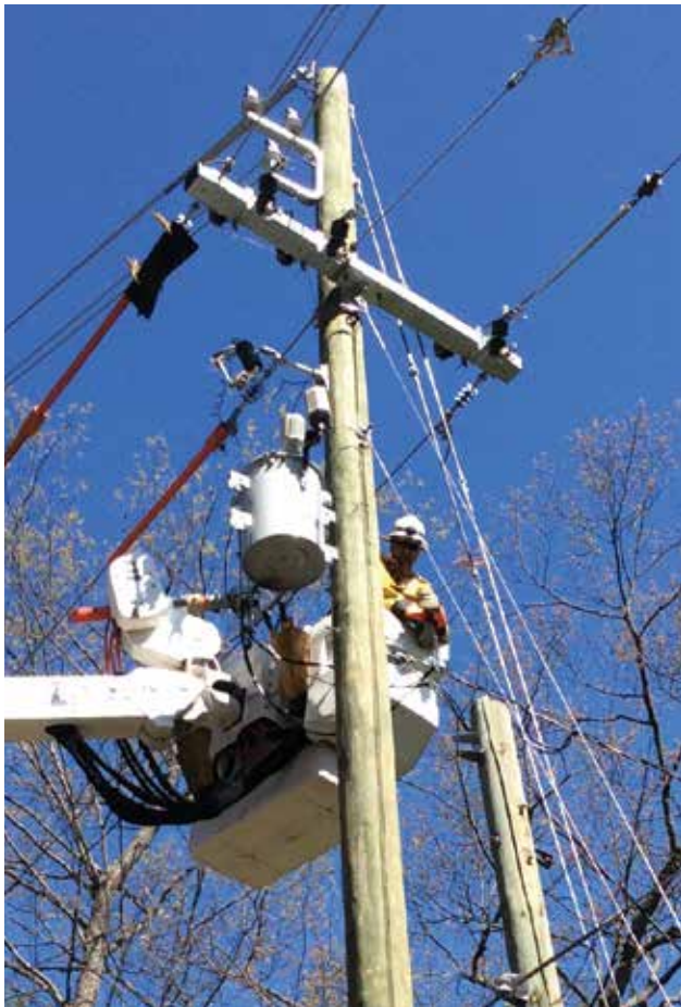
In order for Cherryland to remove old power poles, all cable and telephone wires must be removed as well.
