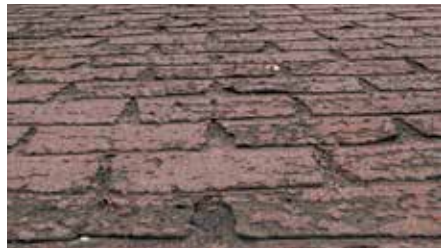
Failed asphalt shingles cracking and peeling.
