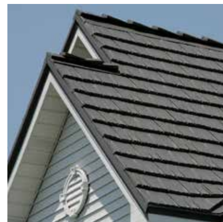
Aluminum shingles from American Metal Roofs.
