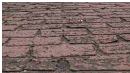
Failed asphalt shingles cracking and peeling.
